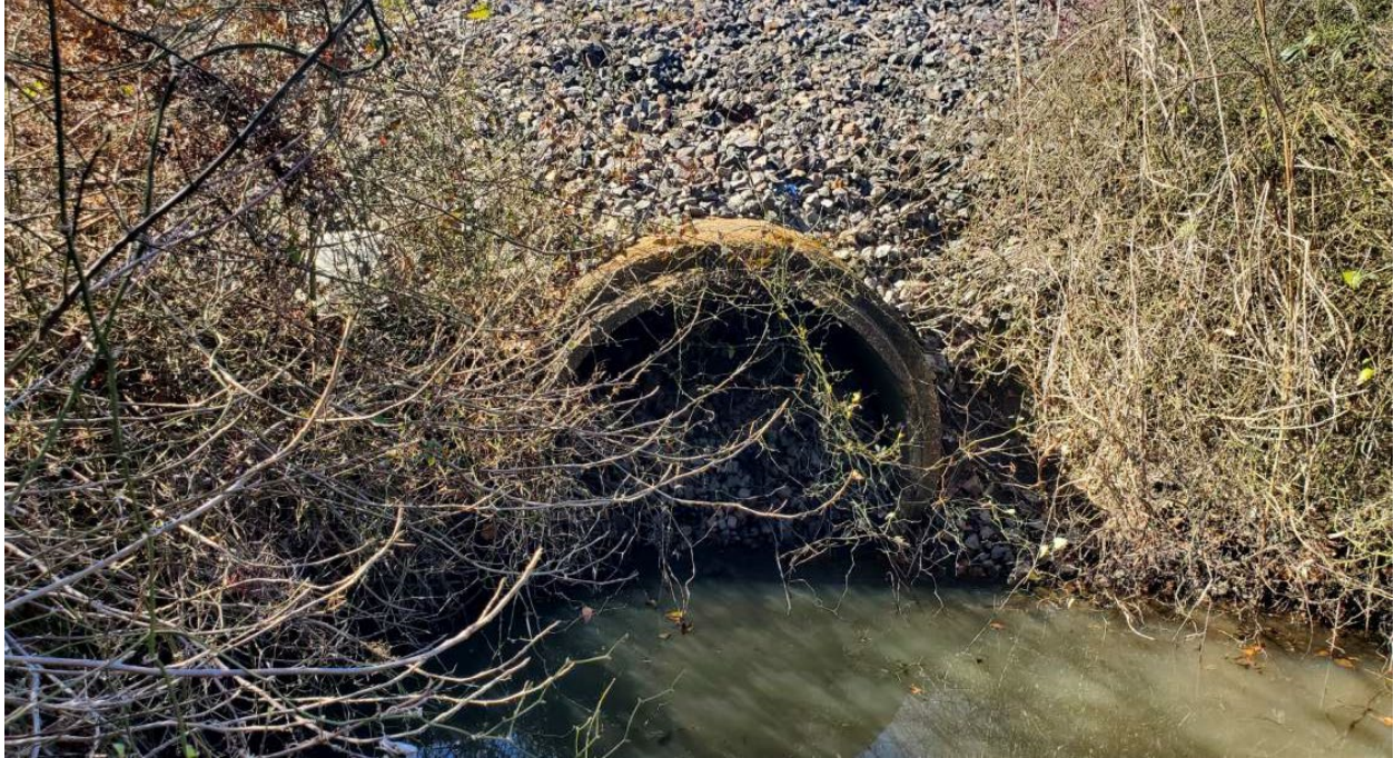
5. Facing south at upstream culvert inlet on north side of rail.
